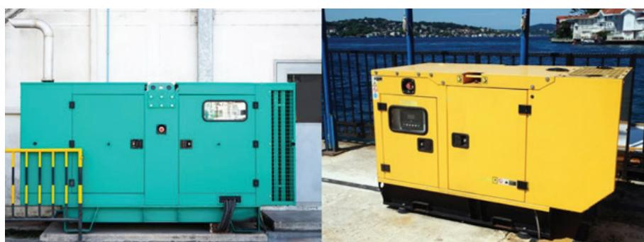
Fig. 4.1.1: DG set mounted on concrete platform
