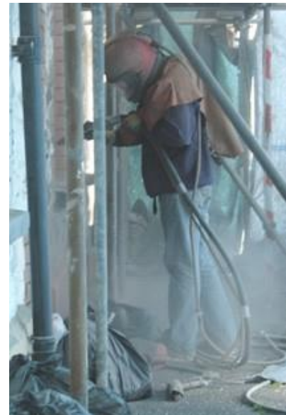
Fig 3.2.4: Abrasive Blasting
