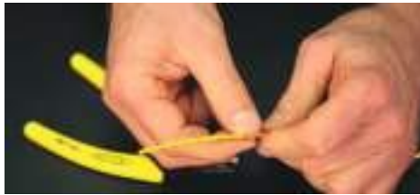
Fig. 3.2.2: Preparing fibre for mechanical splicing
