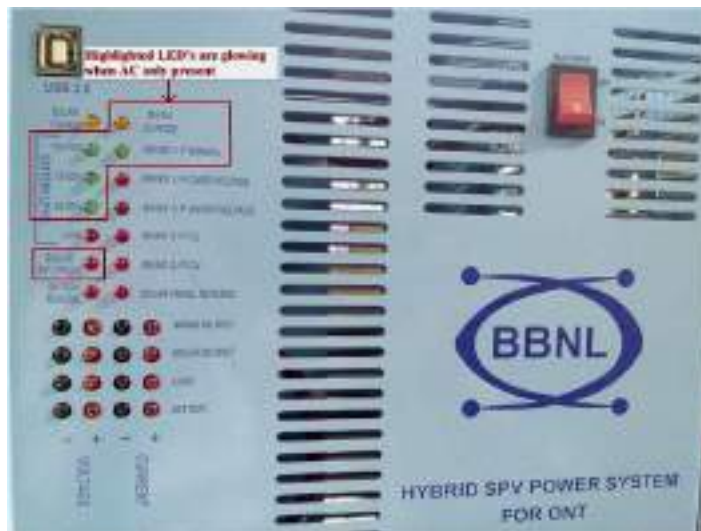
Fig. 7.3.0. Highlighted LED's are glowing when AC only Present
