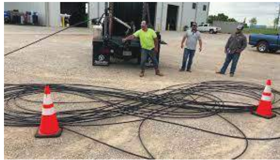
Fig. 2.3.6: Figure 8'ing' of OFC
