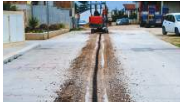
Fig. 2.3.2: Micro-trenching for optical fibre laying
