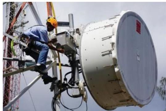
*Fig. 3.1.5: Antenna Alignment*
