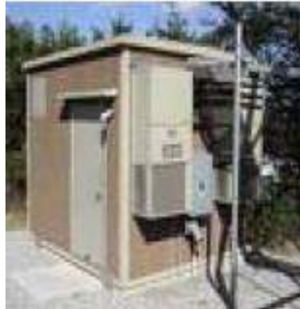
Fig. 2.1.7(i) Concrete Shelter
