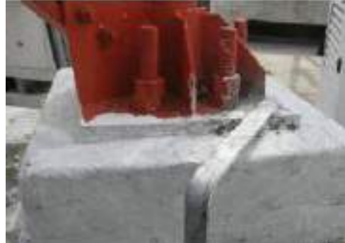
Fig. 2.4.6(ii) Tower earthing with GI strip
