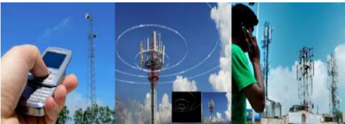
Fig. 1.1.1 Telecom Services in Operation
