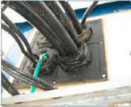
Fig. 2.7.1 Wall Feed Through
