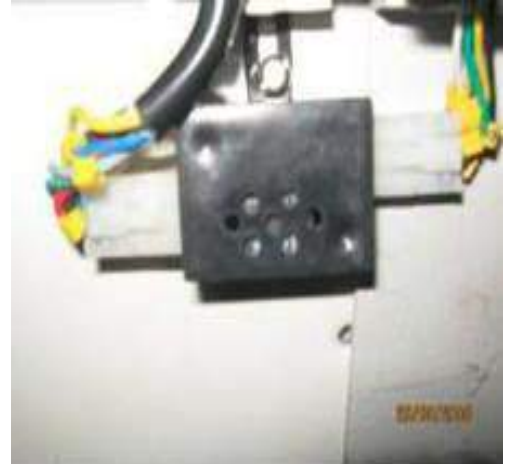
Fig. 2.3.4(ii) Temperature sensor: Present in order to generate Alarm if the temperature raised to the threshold limit.
