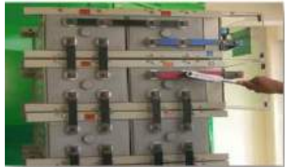
Fig. 2.2.16(ii) Re- torque the terminal bolts once in every six months.
