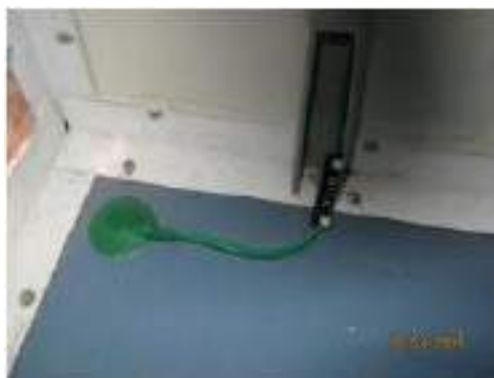
Fig. 2.4.6(iv) Antistatic Grounding
