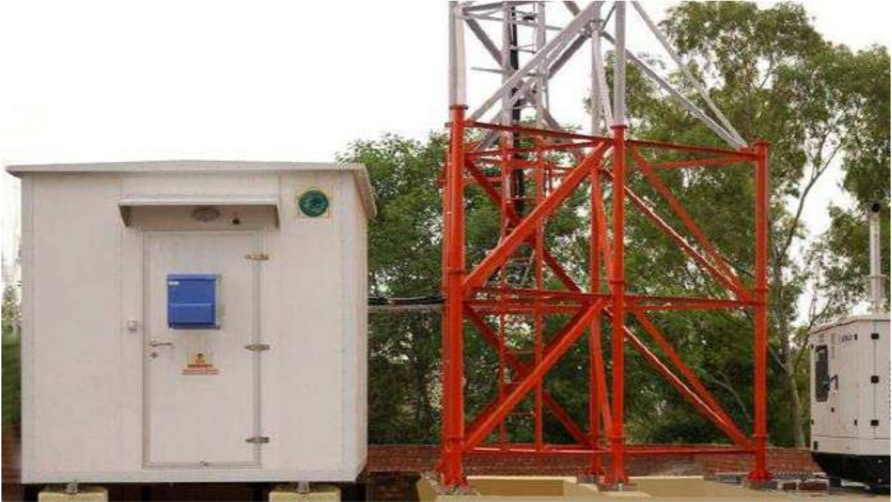
Fig. 2.1.5 Telecom Tower Site
