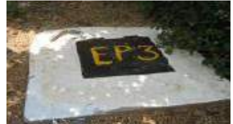
Fig. 2.4.4(i) Three Earthing pits for Tower, Electrical & Electronic equipment.
