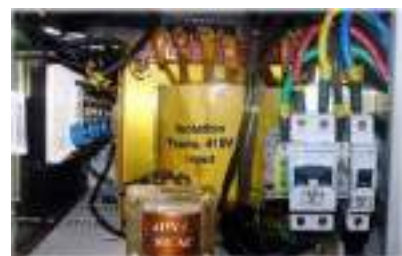
Fig. 2.2.2(vii) Line Conditioner Unit
