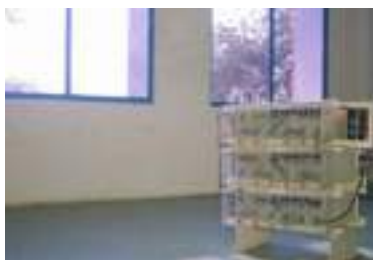
Fig. 2.2.16(viii) Do not allow any direct sunlight to fall on batteries.
