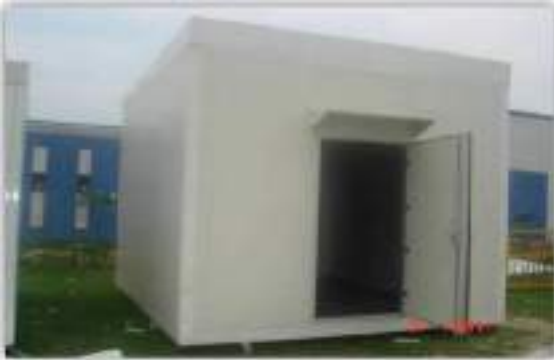
Fig. 2.1.8(iv) Riveted Shelter
