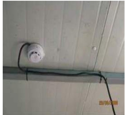
Fig. 2.3.4(ii) Temperature sensor: Present in order to generate Alarm if the temperature raised to the threshold limit.
