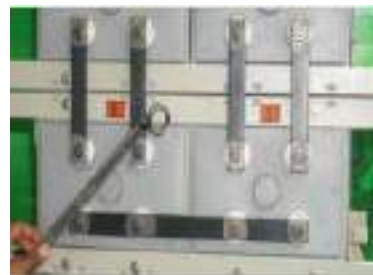
Fig. 2.2.16(viii) Do not allow any metal objects to fall across the battery terminals.
