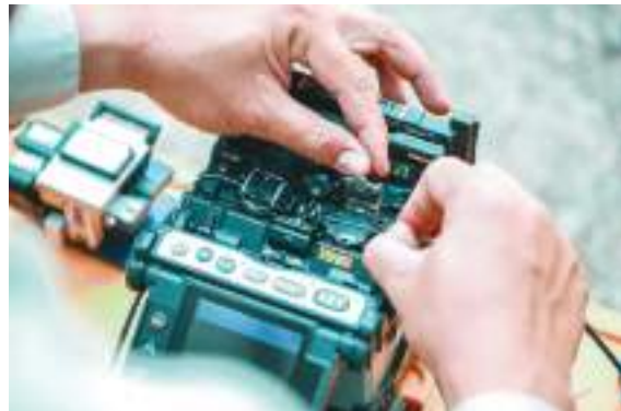
Fig. 1.2.3: Splicing of Optical Fibre
