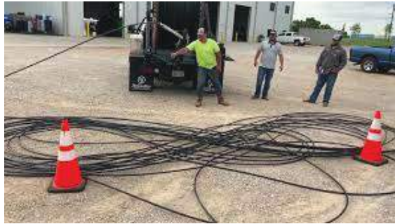
Fig. 2.3.6: Figure 8'ing' of OFC
