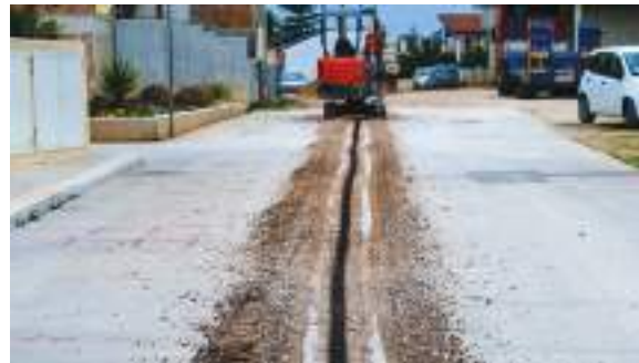
Fig. 2.3.2: Micro-trenching for optical fibre laying
